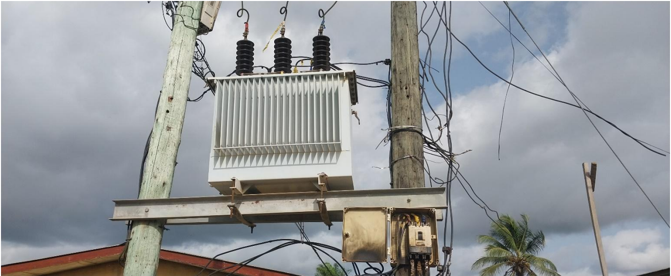
Damaged Transformer Breaker Enclosure
