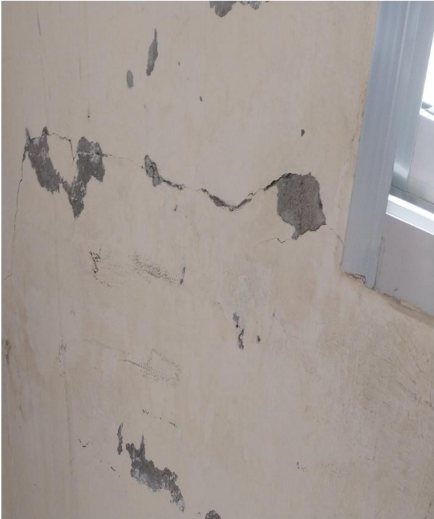
Crack on Stockton Creek Control Building
