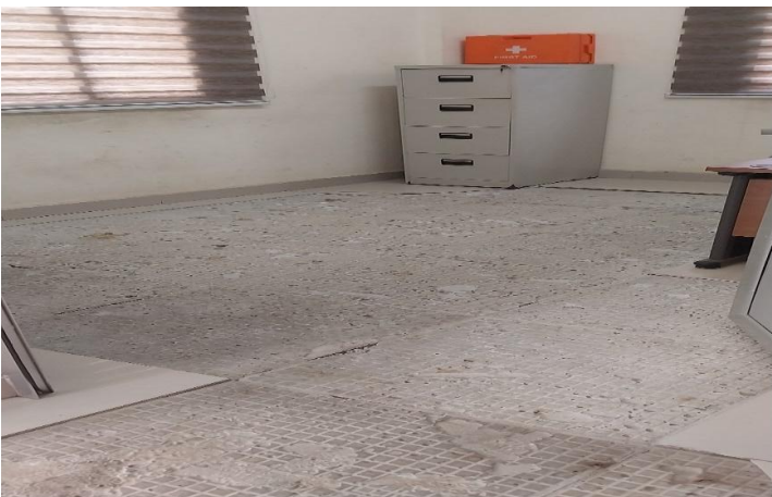
Damaged Floor/Tiles in Stockton Creek Control Room
