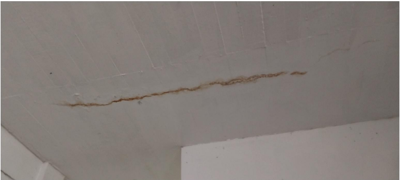
Leakage Roof Slab in Control Room
