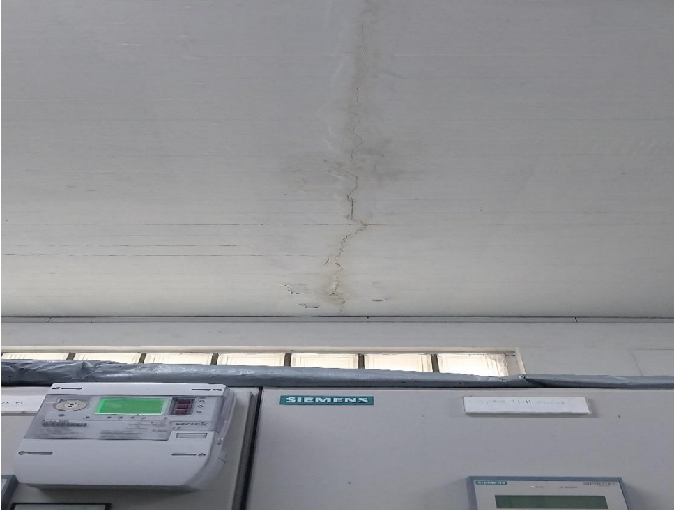
Leakage Over 22 kV Switchgear
