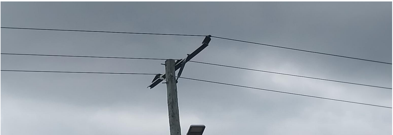
Leaning Cross-arm with Insulator on the Somalia Drive on Gardnerville - Stockton Creek Feeder
