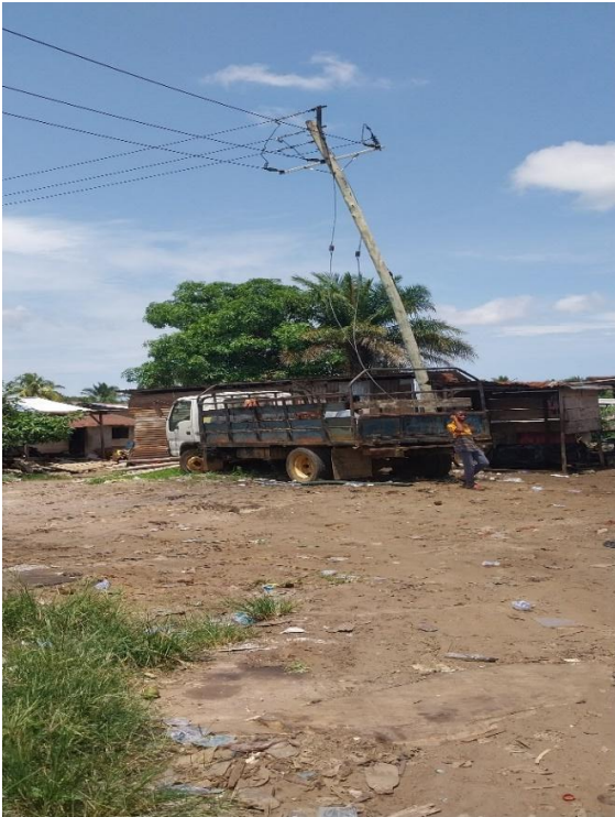
Leaning MV Pole from Diverted Lines from the Main Somalia Drive
