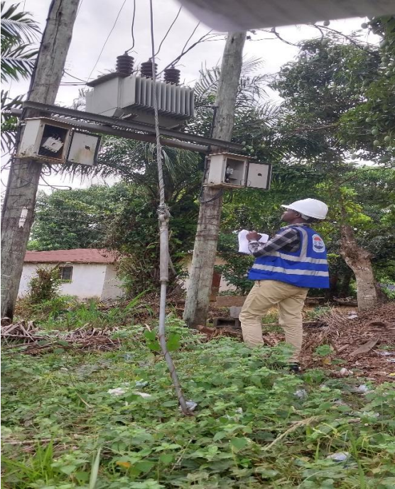
Damaged Transformer Breaker Enclosures
