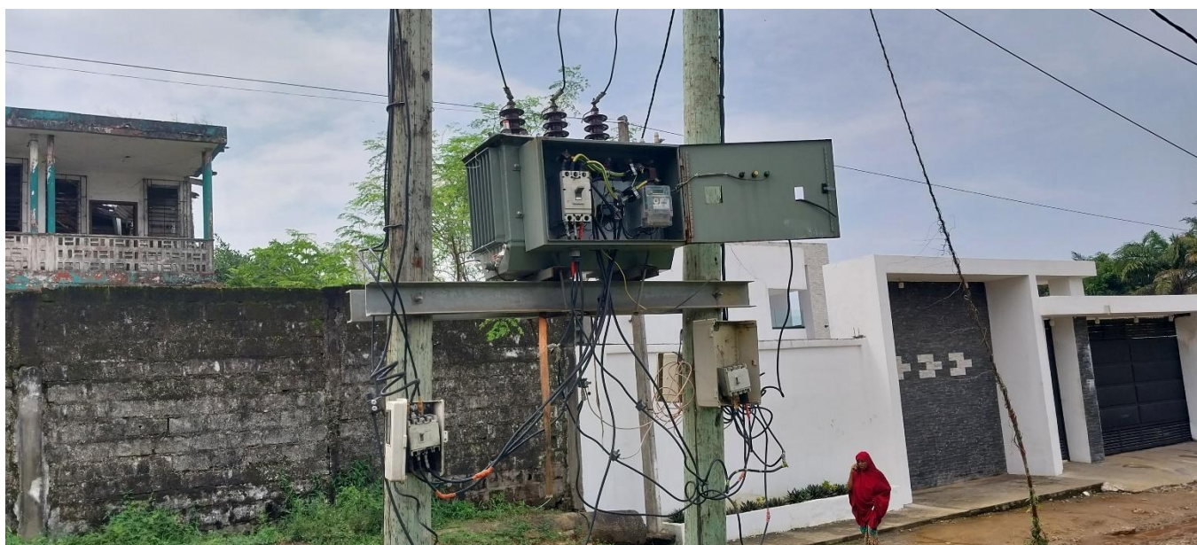
Damaged Transformer Breaker Enclosures
