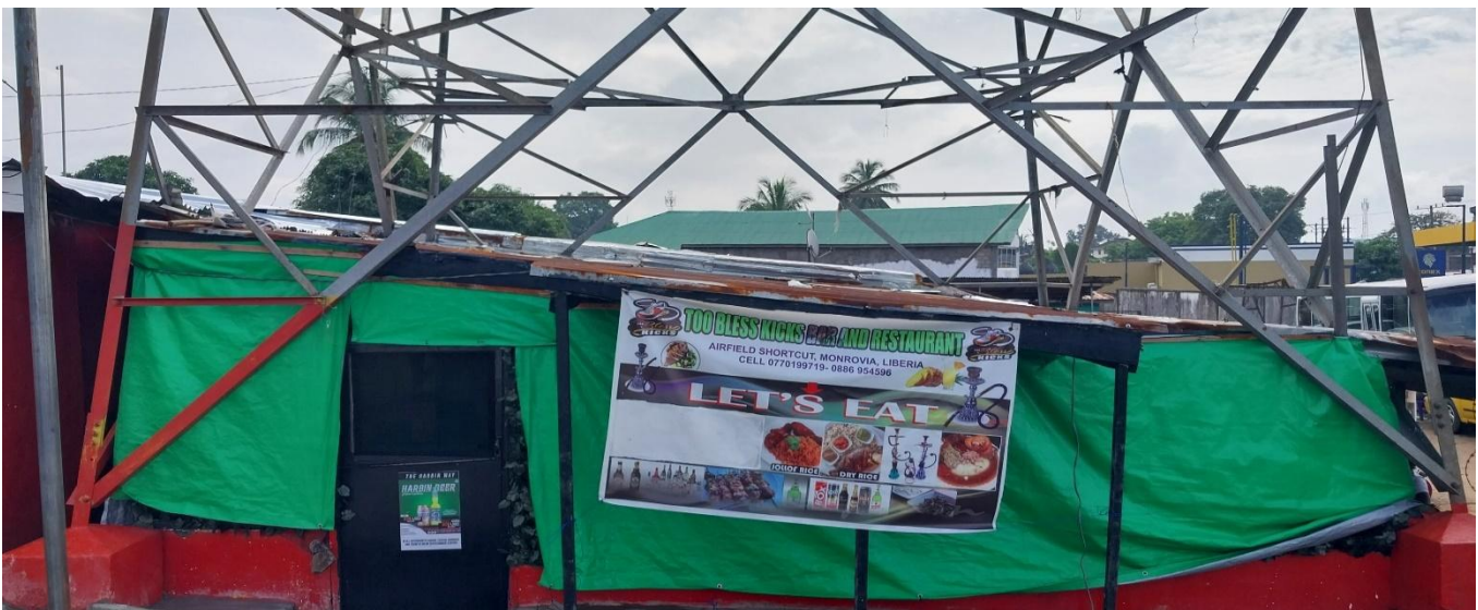
Structure Built in Tower Footing along Airfield Short Cut
