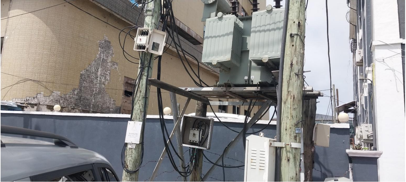
Damaged Transformer Breaker Enclosures
