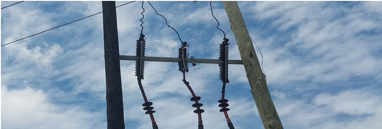
Middle Phase of Cut-Out Fuse Bypassed at Gardnerville Substation
