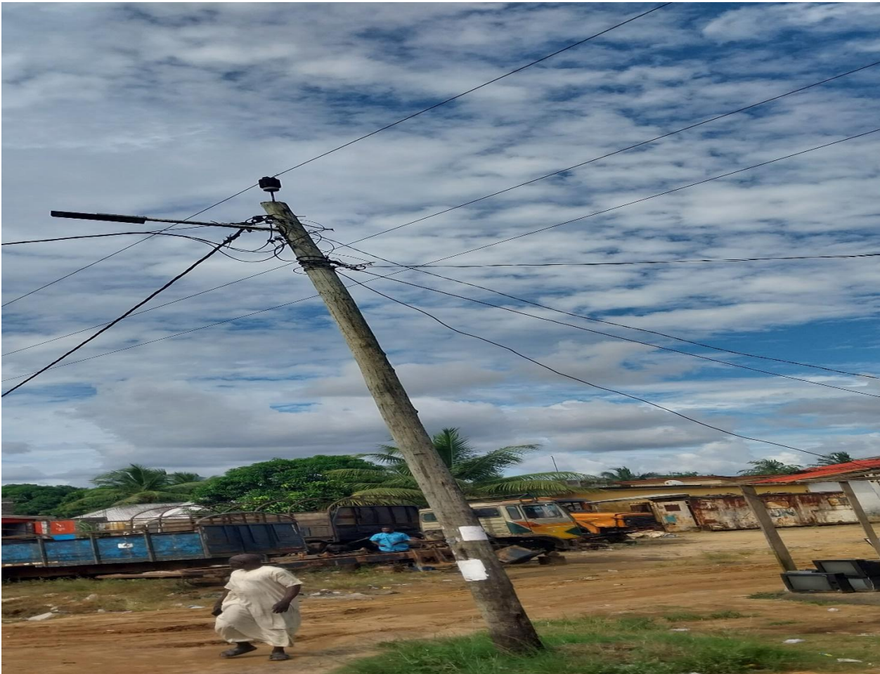
Leaning LV Pole with Insulator at the Top of the Pole
