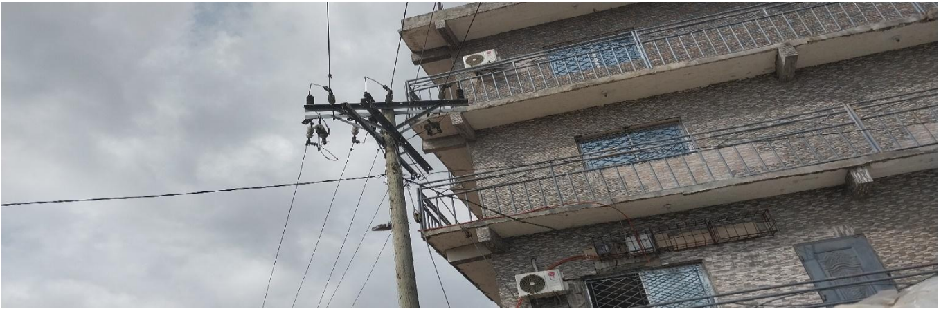
MV Very Close to Structure
