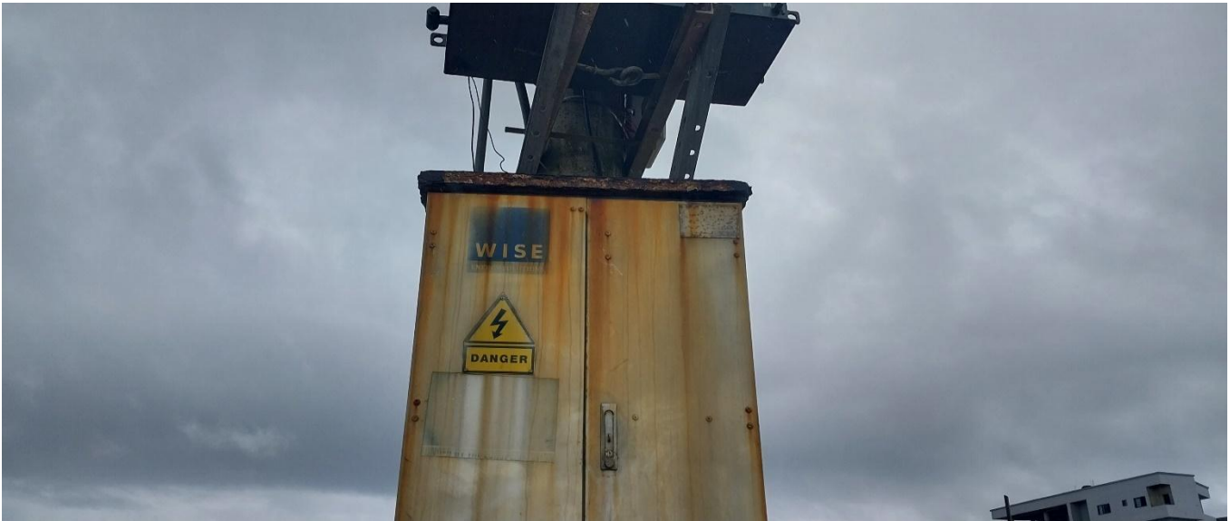
Rusting Low-Voltage Distribution Box Along the Coastal Belt
