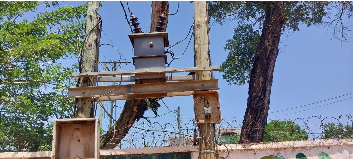
Damaged Transformer Breaker at LBS
