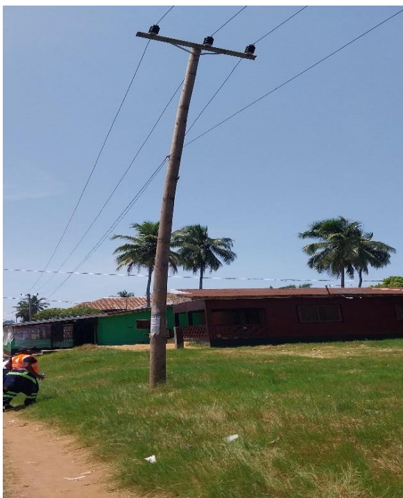
Leaning MV Pole at the Back of Kool FM
