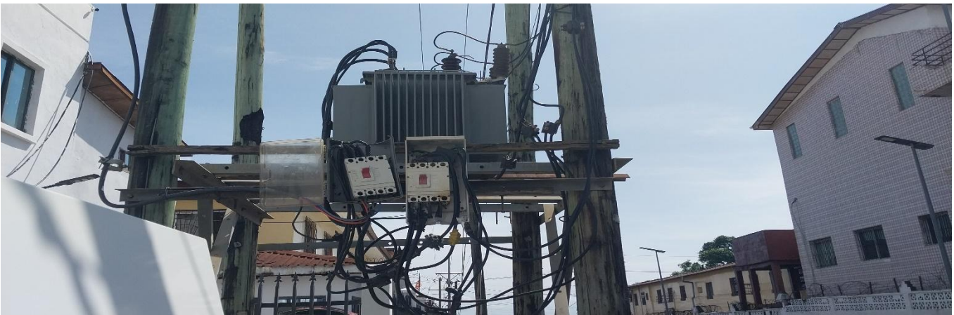
Damaged Transformer Breaker Enclosures
