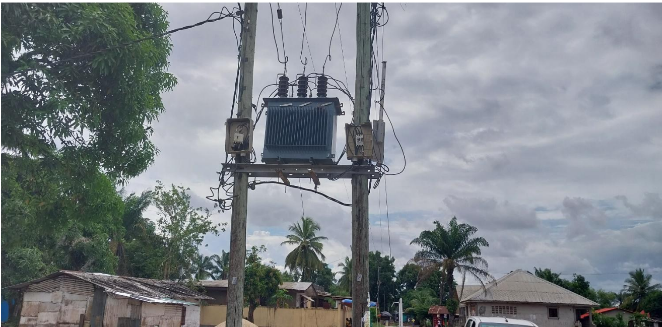
Badly Leaning Transformer with Damaged Transformer Breaker Enclosures
