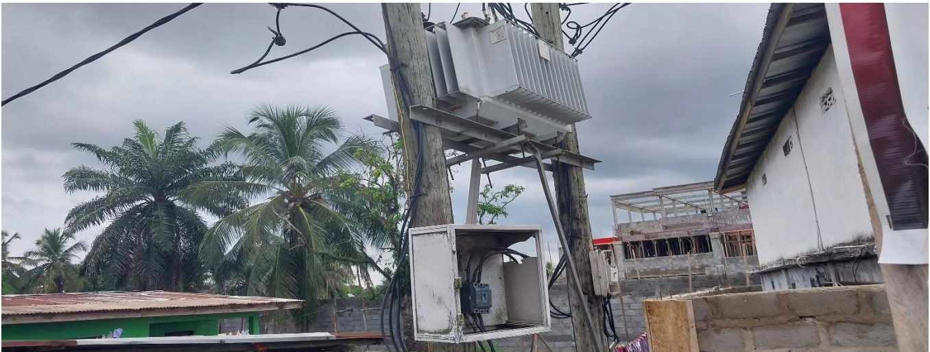
Damaged Enclosures
